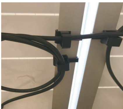
Outside the frame, wiring in cross.
