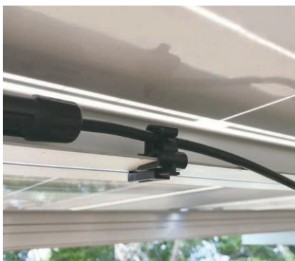
Inside the frame, wiring in parallel.
