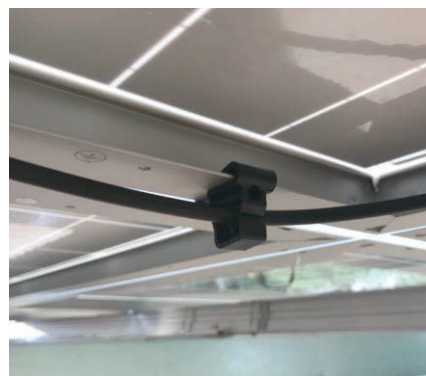
Outside the frame, wiring in parallel.
