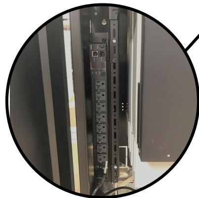
1 UR Vertical Patch o PDU
