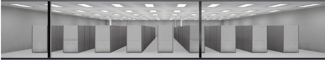
Figure 3. Baseline Model of a Data Center with White Cabinets.
