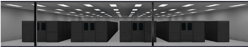
Figure 5. Model of a Data Center with Black Cabinets and Black Cold Aisle Containment.
