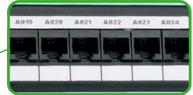
Patch Panel / Face Plate Labels
