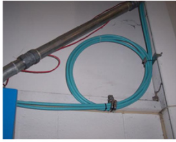
Figure 13 Coiled Slack Loop
