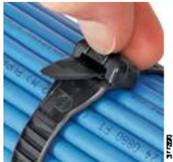
Figure 25 Elastomeric Ties for Bundling Fiber
